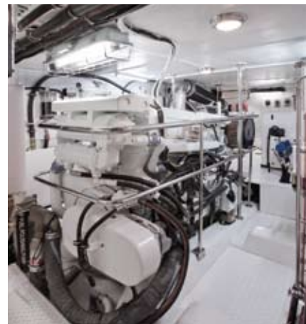
Stainless-steel rails surround the Lugger main engine, which is positioned for 360-degree access.
